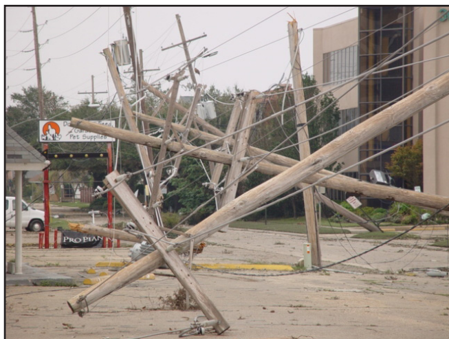
Downed power lines on Causeway and Esplanade in New Orleans after Hurricane Katrina, August 2005.
